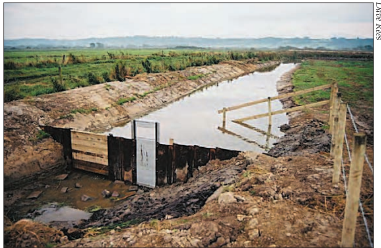
Plate 7.7 Completed trench sheet sluice.
