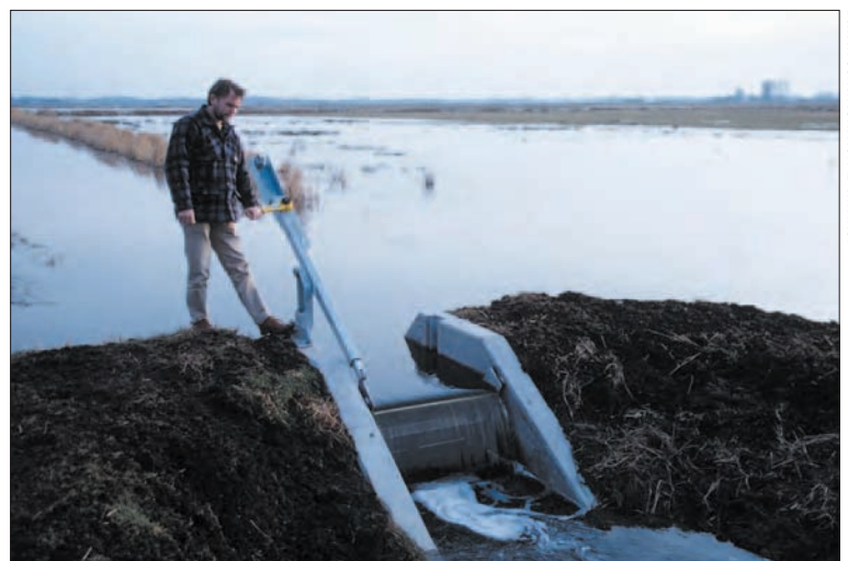
Plate 7.20 Regulating of natural water levels by adjustable weirs in the fens at Lake Dümmer.
