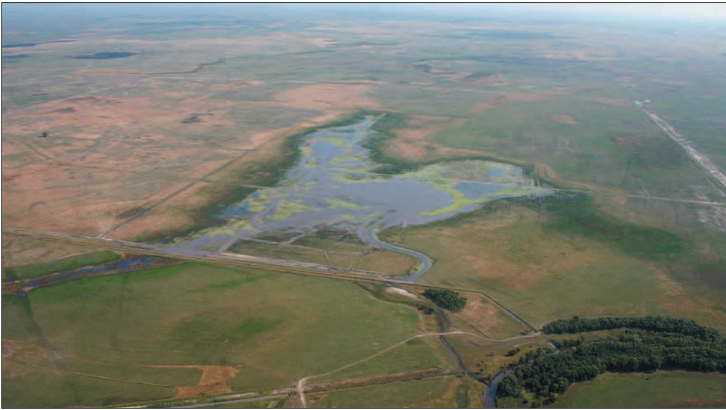
Plate 7.18 The flooded marsh after the completed works.
