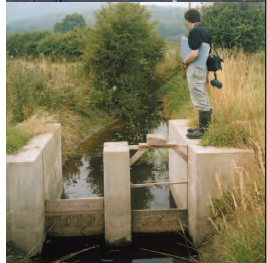
Plates 5.12–5.13 Pipe sluice (top) Dropboard sluice (bottom)
